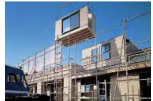
Swift on-site assembly completed in just one day
