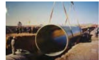
Reinforced plastic compound pipe installation
