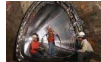
SPR method, which allows pipe restoration without excavation.
