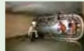
A sewage pipe renewal (SPR) system that reduces waste by eliminating the need to open new trenches in roads
